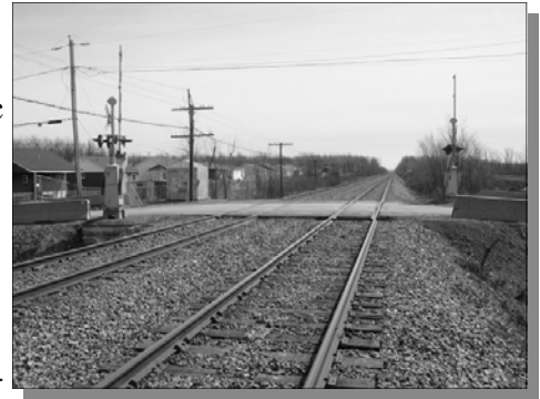
The “Texas” crossing slated for widening
