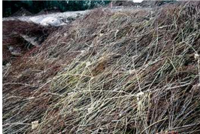
Figure 26: Brush Mat Re-Vegetation Technique
