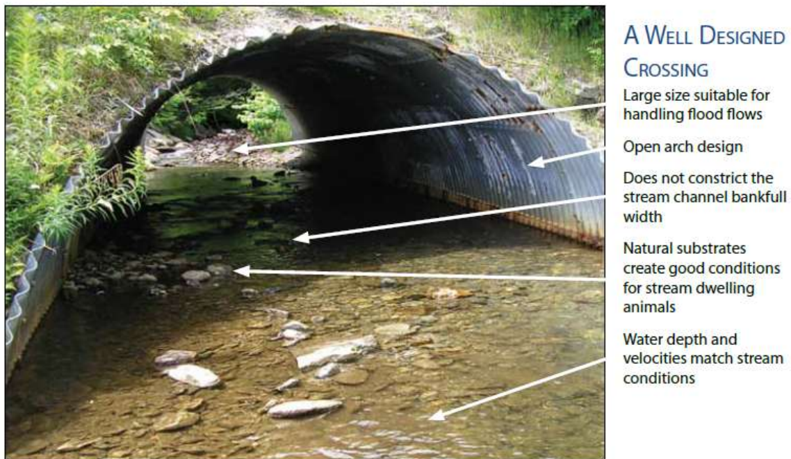
Figure 13: Characteristics of a Well-Designed Creek Crossing
