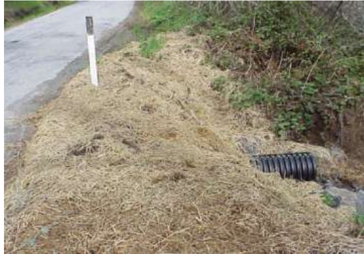
Figure 18: Mulching Slopes with Loose Straw to Reduce Erosion
