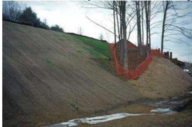
Figure 19: Using Coir Mats to Protect Exposed Areas Prior to Re-vegetation
