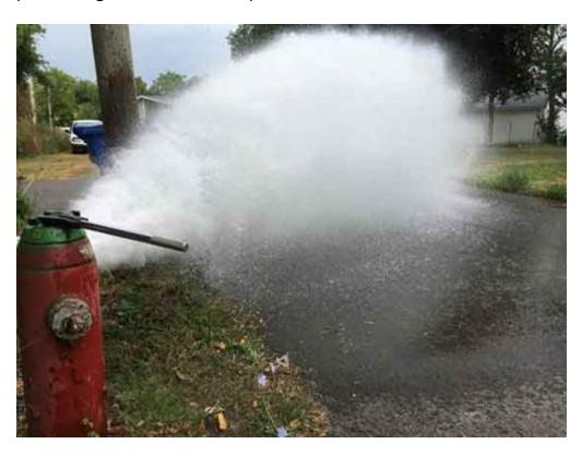
Unidirectional Flushing is the process of cleaning the water system by flowing water in one direction through the mains. This is accomplished by closing specified valves and by flushing strategically located hydrants.
